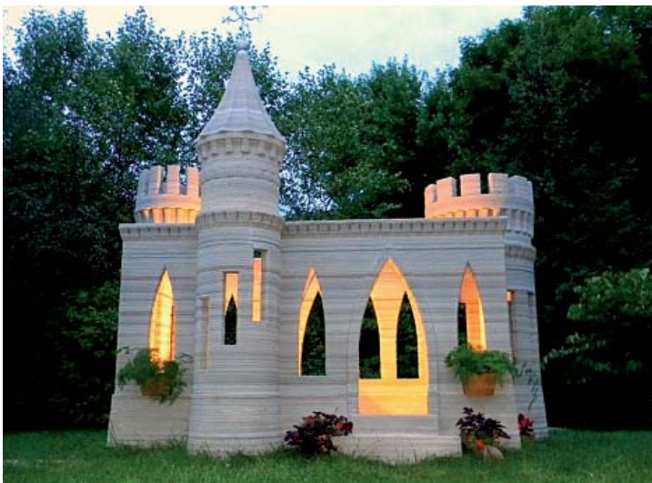
Printani betonski dvorac; Izvor fotografije: https://www.concreteconstruction.net/business/technology/3d-printed-concrete-the-future-is-here_c
